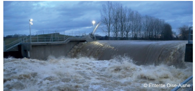
Flap gates at the Proisy site in operation in 2011
