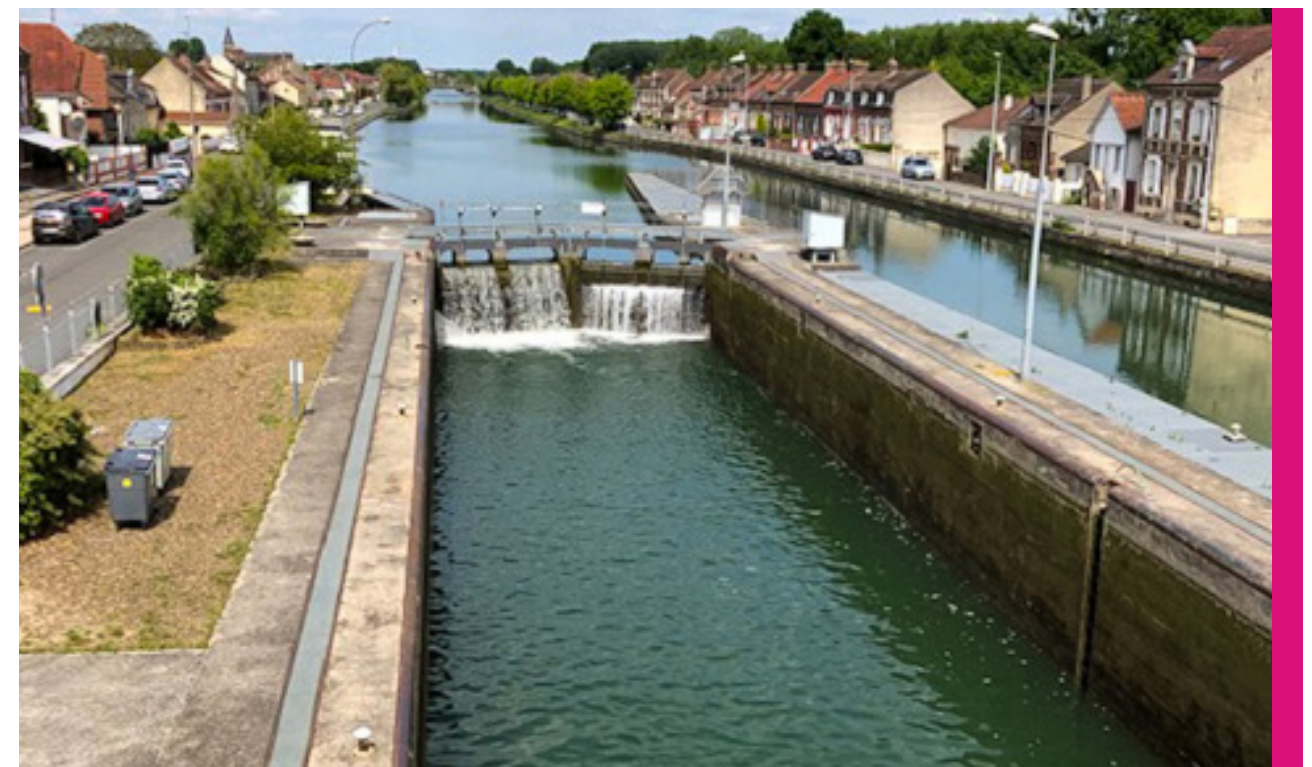
Above: Lock in action on the Oise River
